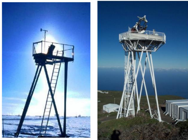
Figure 22. 7.5-meter tower at the South Pole (left). 15-meter tower for DOT at La Palma, Spain (right) [9].
