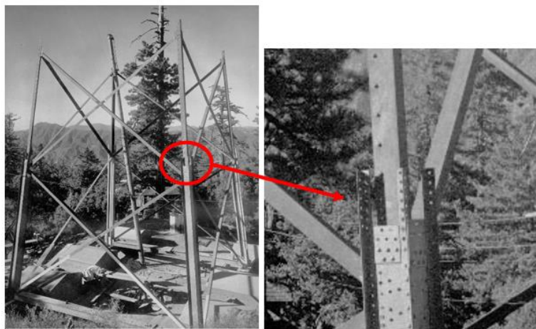
Figure 25. Highlighting the inner and outer tower of the 150-Foot Solar Tower at Mt. Wilson, CA [12].
